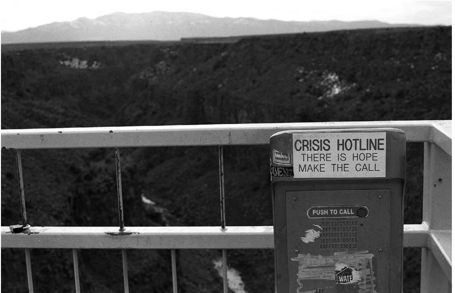
Rio Grande Gorge Bridge, Taos, New Mexico – Mitch Marty
